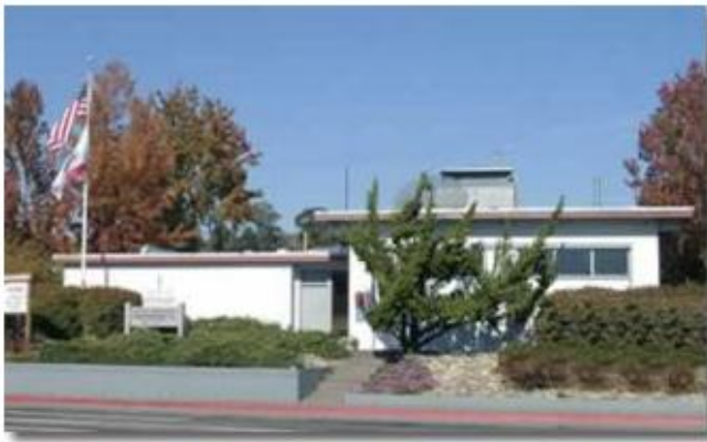
Fire Station 2 210 Third Street San Rafael, CA 94901
